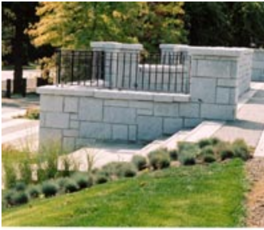
Hollybridge Pumpstation - Middle Arm Trail staging area
