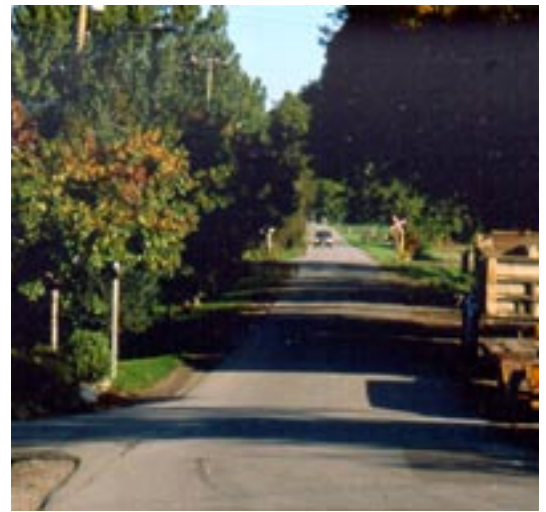
No. 4 Road - South Dyke
