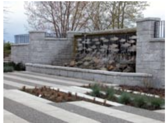
Hollybridge Way pump station
