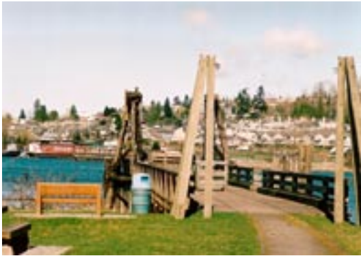
No. 7 Road Pier (former CNR barge loading pier)
