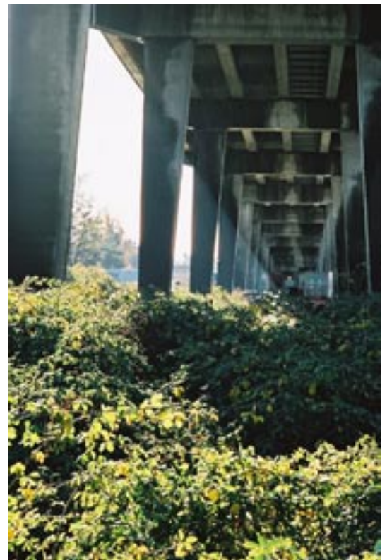
Knight Street bridge
