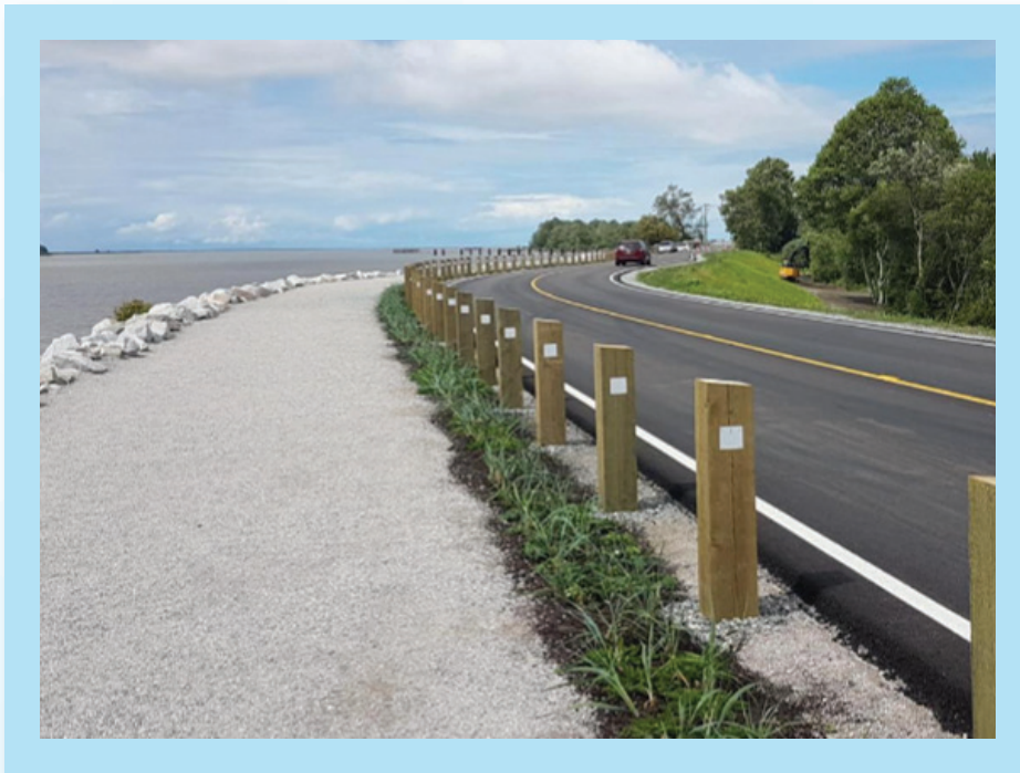
The City successfully upgraded 650 m of dike along the Fraser River's south arm between Gilbert Road and No. 3 Road. This upgrade raised the dike by approximately 1.5 m and included a multi-use trail separated from traffic lanes and incorporated seating, picnic areas and arrival points with wayfinding and parking.
