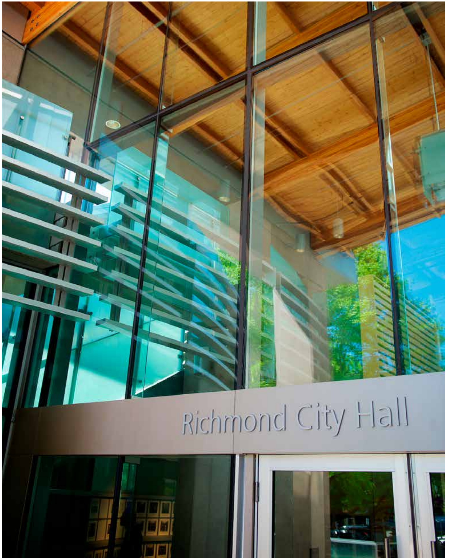
Sustainability has always been an important City initiative. The current City Hall, which was officially opened in May 2000, was ahead of its time with its advanced technology and energy efficient and environmentally-sensitive design.
