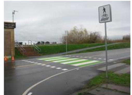
New Ramp to the Middle Arm Dyke Trail at River Road
