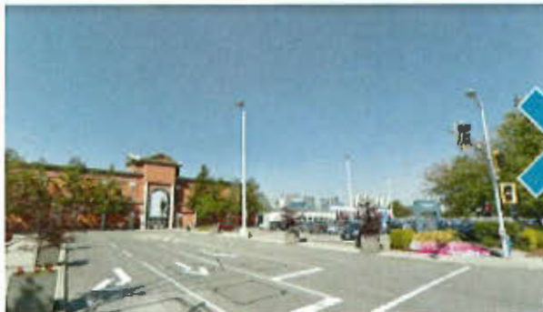
Existing Park Road
