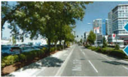
No 3 Road - Existing condition
