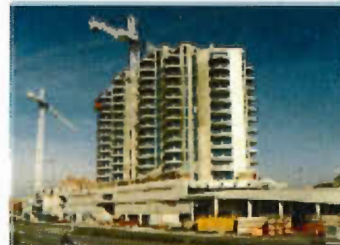
1996 RICHMOND POPULATION 143,000 Construction of Horizons Towers brings residential units to Centre
