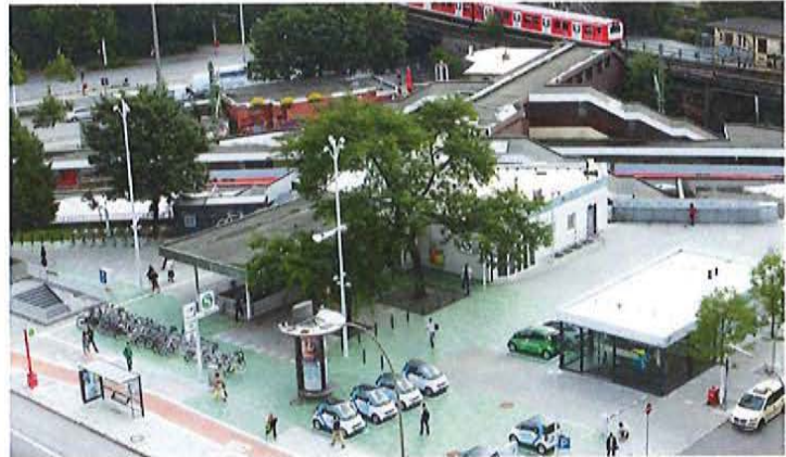
Clustered, street-level transportation amenities. Source: Hamburger Hochbahn AG
