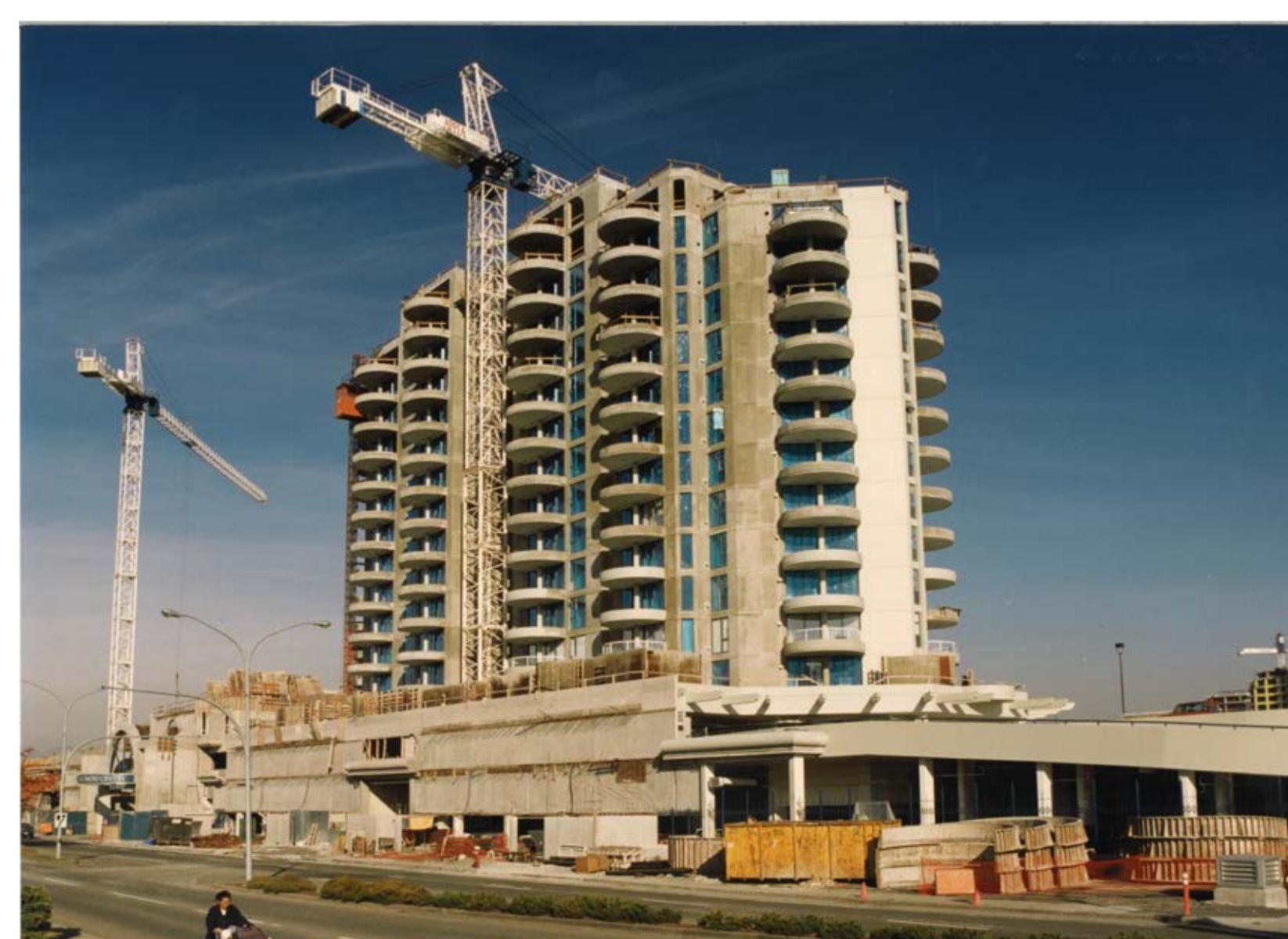
1996 RICHMOND POPULATION 149,000 Construction of Horizons Towers brings residential units to Centre
