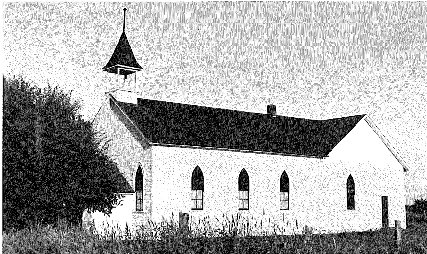
④ The South Arm United Church building in 1930. At this time it was being used as a "summer centre."
