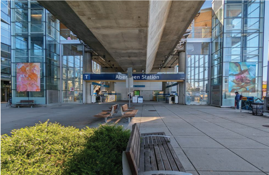
Figure 1. Cherry Archer, Membranes & Pith 305 & Reverie 25 , Aberdeen Canada Line Station
