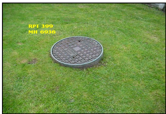
Outside Manhole Photograph
