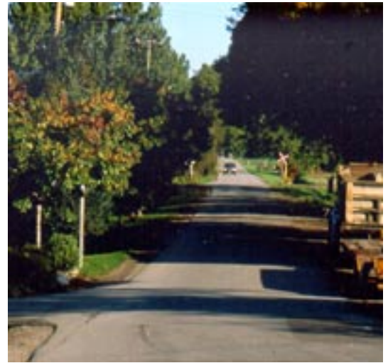
No. 4 Road - South Dyke
