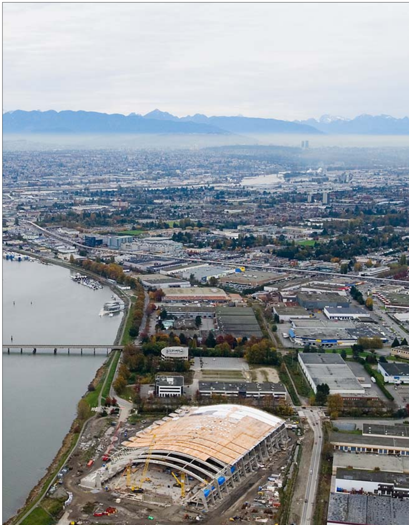
Aerial view of City Centre, June 2007, showing Richmond Oval and Canada Line under construction.
