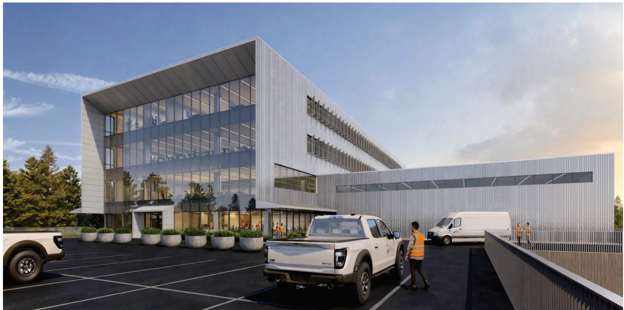
Northwest View – From Fleet Parking on Level 1
