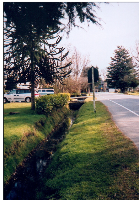
Streetscape with 6 meter roadway, ditch and monkey puzzle tree
