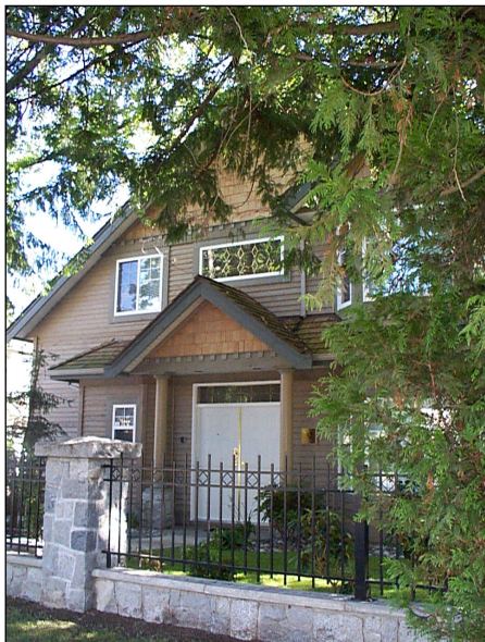
Prominent Building Entrance
