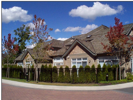
Secondary Roof Elements
